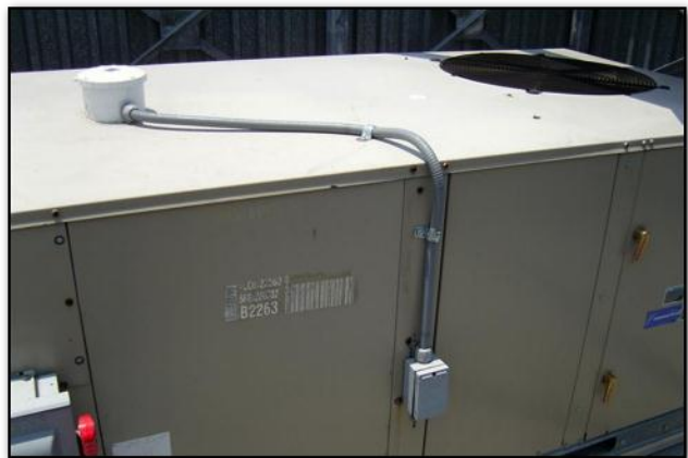
Because the redesigned X-Plus fixture from UV Resources can be easily mounted from the exterior of any HVAC system, air handler, plenum or duct, the NEMA rated fixture is ideal for hard-to-access outdoor and indoor equipment.
